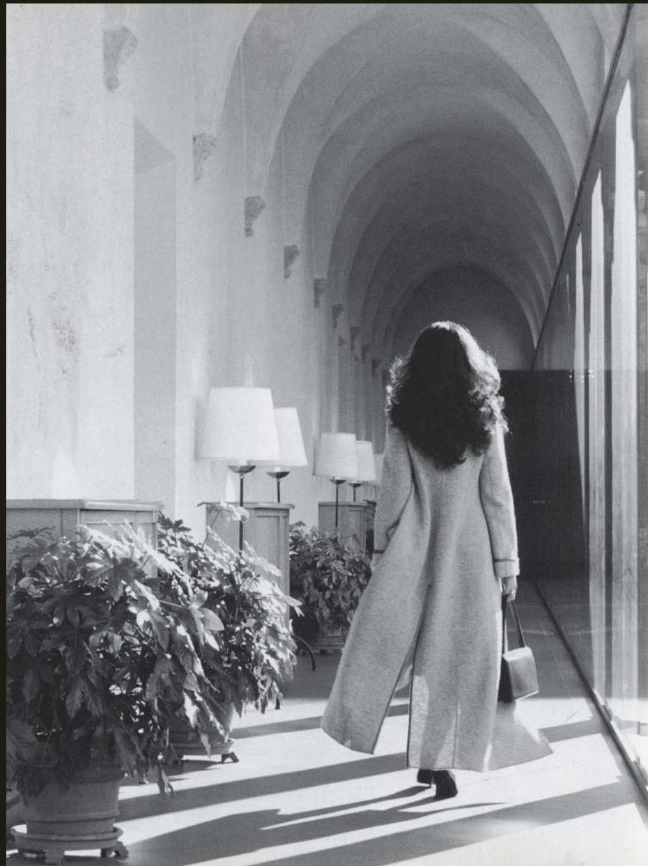
limestone & plastered groin vaults
